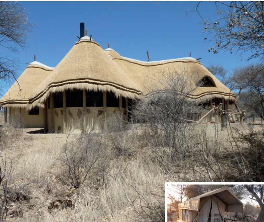
Central building (above) and two-person tent of a field research station Biosphere Expeditions has helped put in place in Namibia
